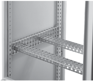
Grid Strap installation (side to side)
